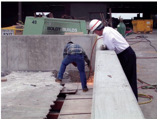
Fig. 21 – Detensioning Tendons by Heating with a Torch
