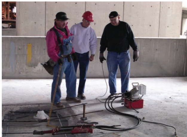
Fig. 11 – Stressing of Tendon at Intermediate Stressing Anchor
