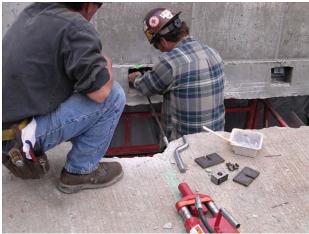
Fig. 19 – Installation of Split Anchors
