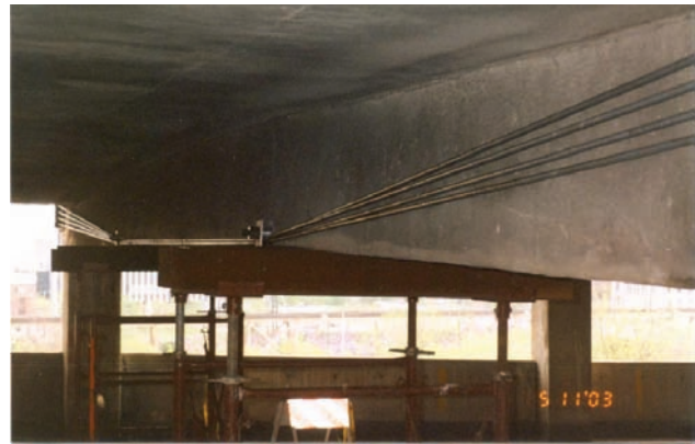
Fig. 27 – Deviated Beam Strengthening Tendons
