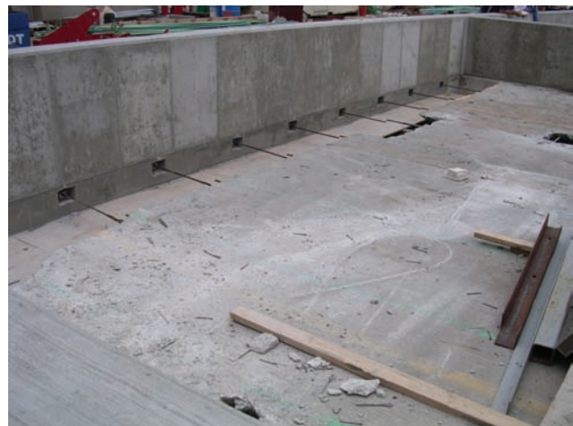
Fig. 18 – New Perimeter Beam at the Edge of Opening
