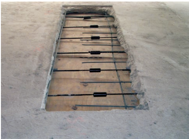
Fig. 9 – Couplers for Slab Repair
